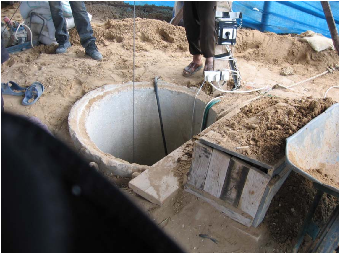
Picture 25: One of the tunnels seen by the Committee.
