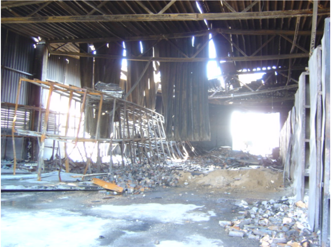
Picture 14: The destroyed UNRWA warehouse.
