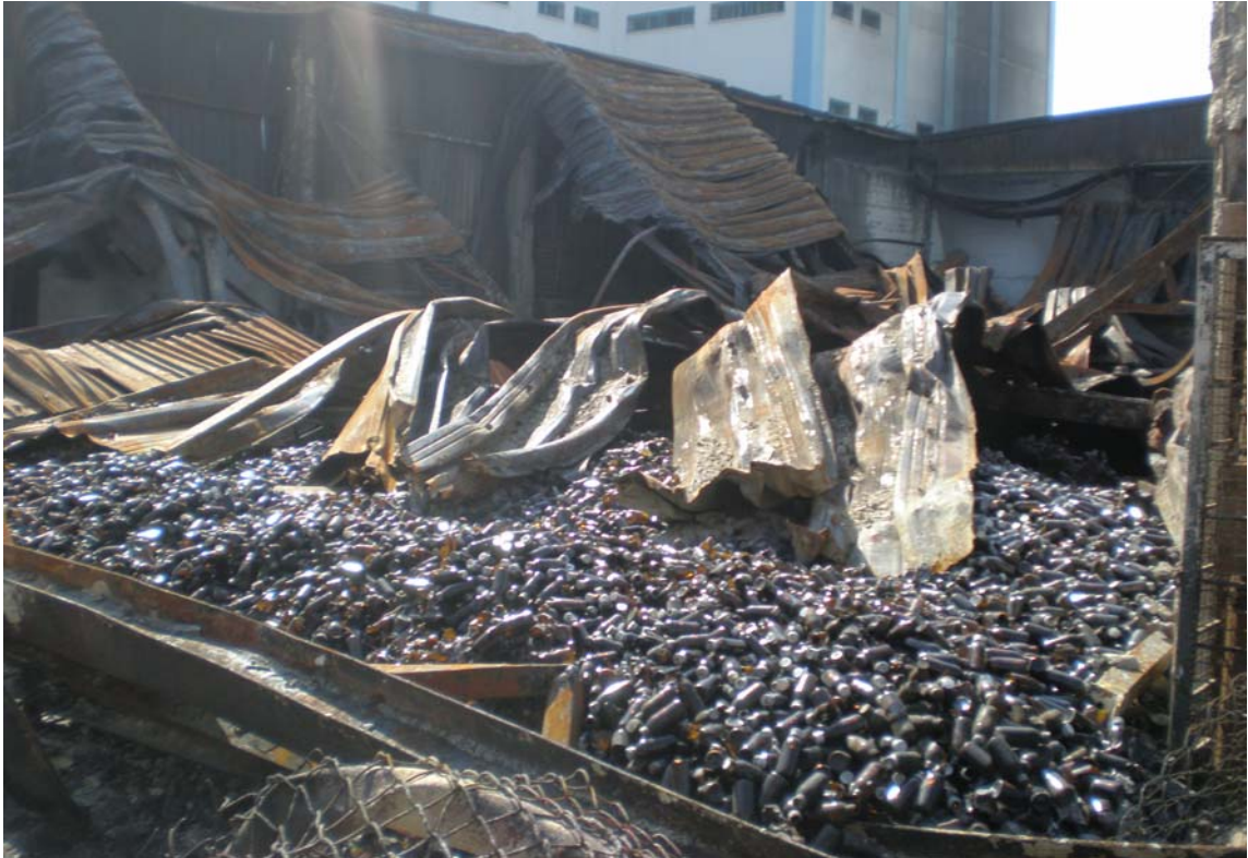
Picture 15: The destroyed UNRWA warehouse.
