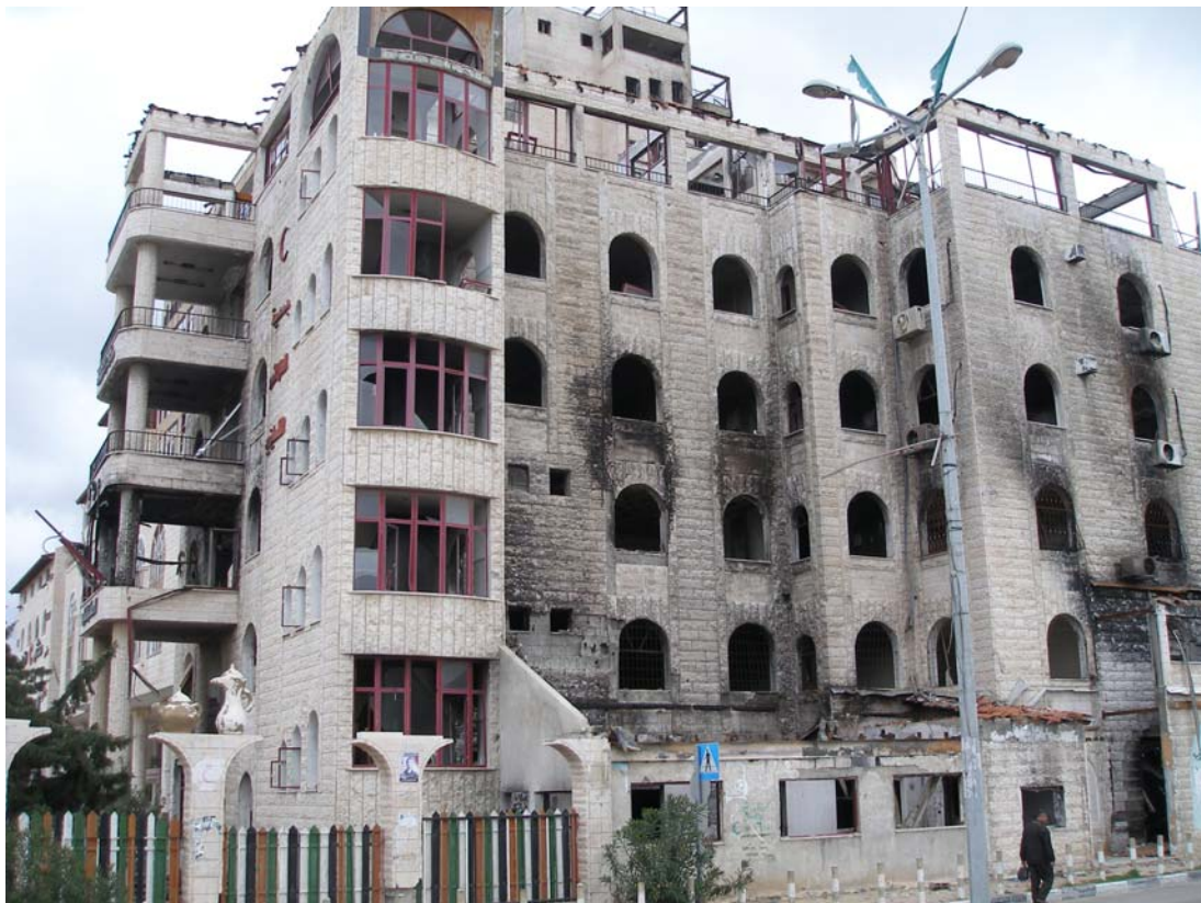
Picture 7: Damage to the Al-Quds Hospital.
