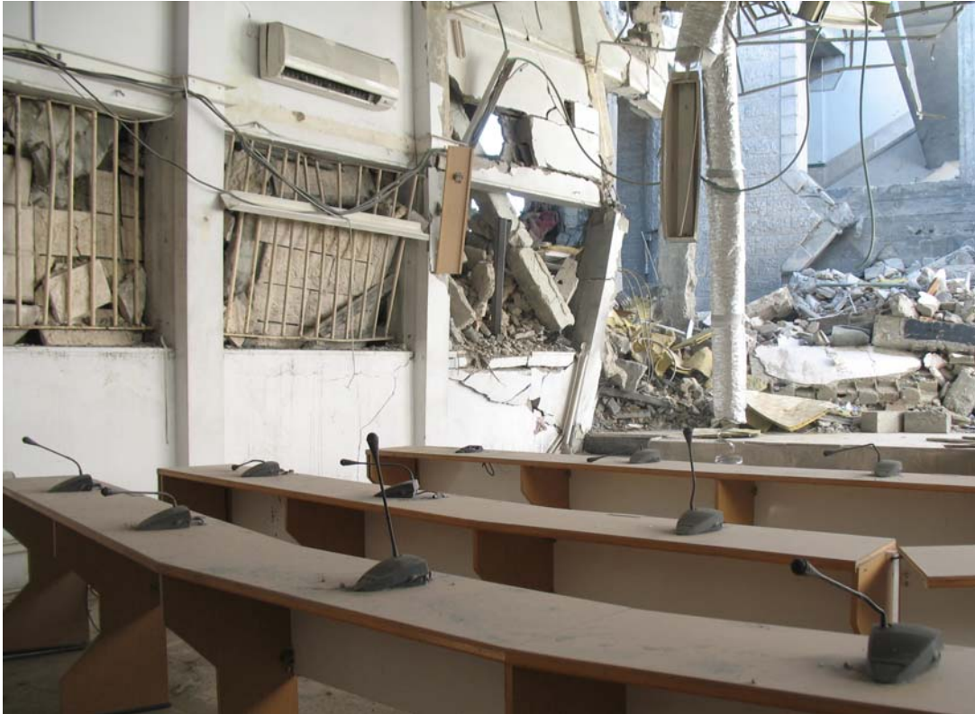
Picture 17: The destroyed parliament building, showing where joint sittings were formerly held.
